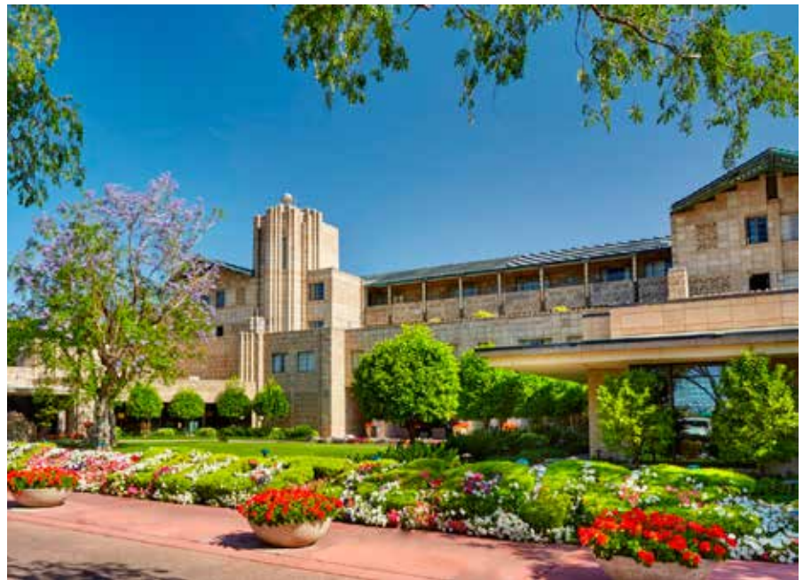
The Arizona Biltmore Waldorf Astoria Resort in Phoenix, Arizona, has made extensive customizations to building and response codes in the software that guide staff through the collection of incident information at the scene.
